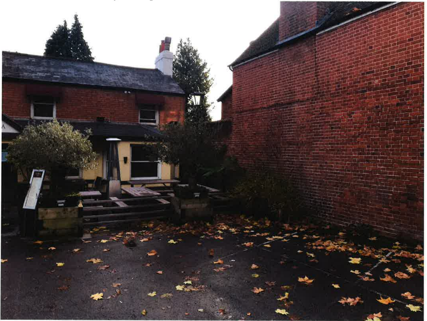
Picture 3 Side of Crossways Cottage
