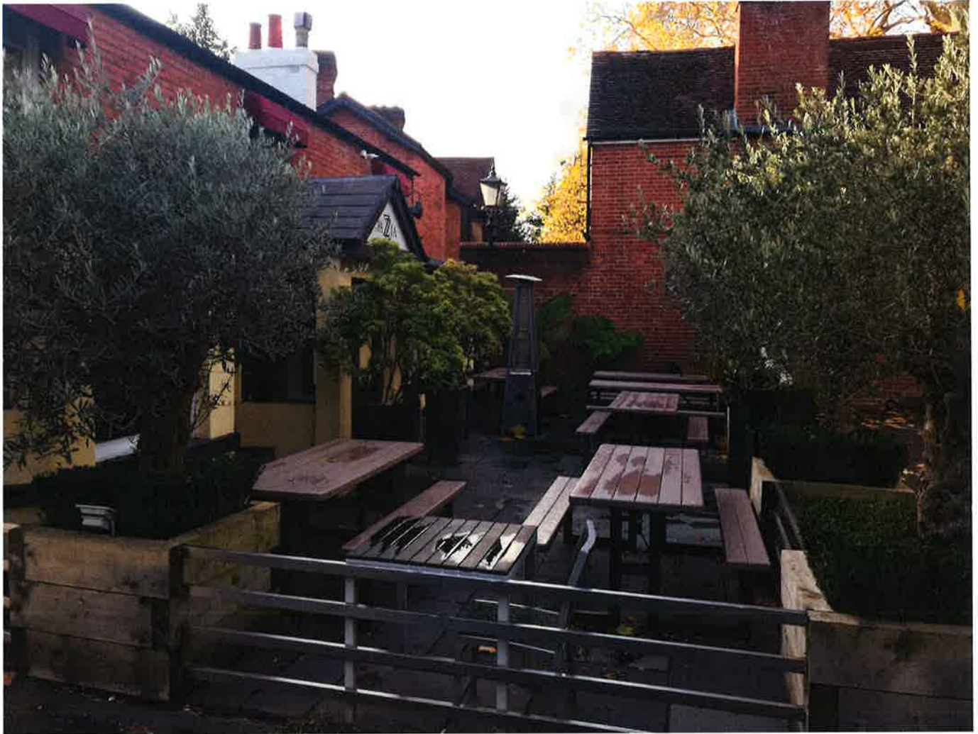
View of from of Pazzia Restaurant looking towards the side wall of Crossways Cottage. The external tables are not shown on the licensing plan and are under the rear bedroom window of Crossways Cottage
